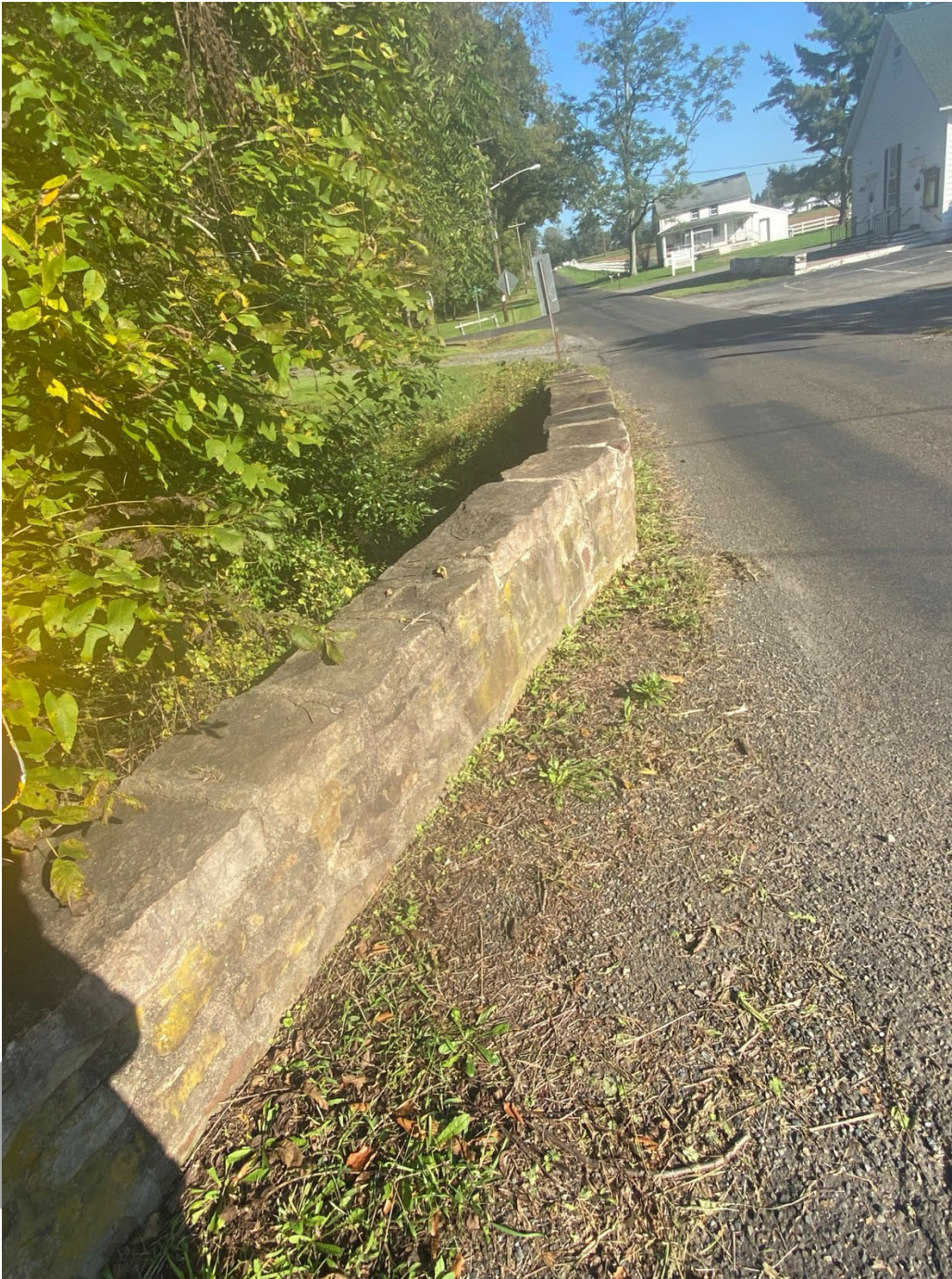
Photo 8: West (upstream) wingwalls and parapet, view facing north showing the capstones.
