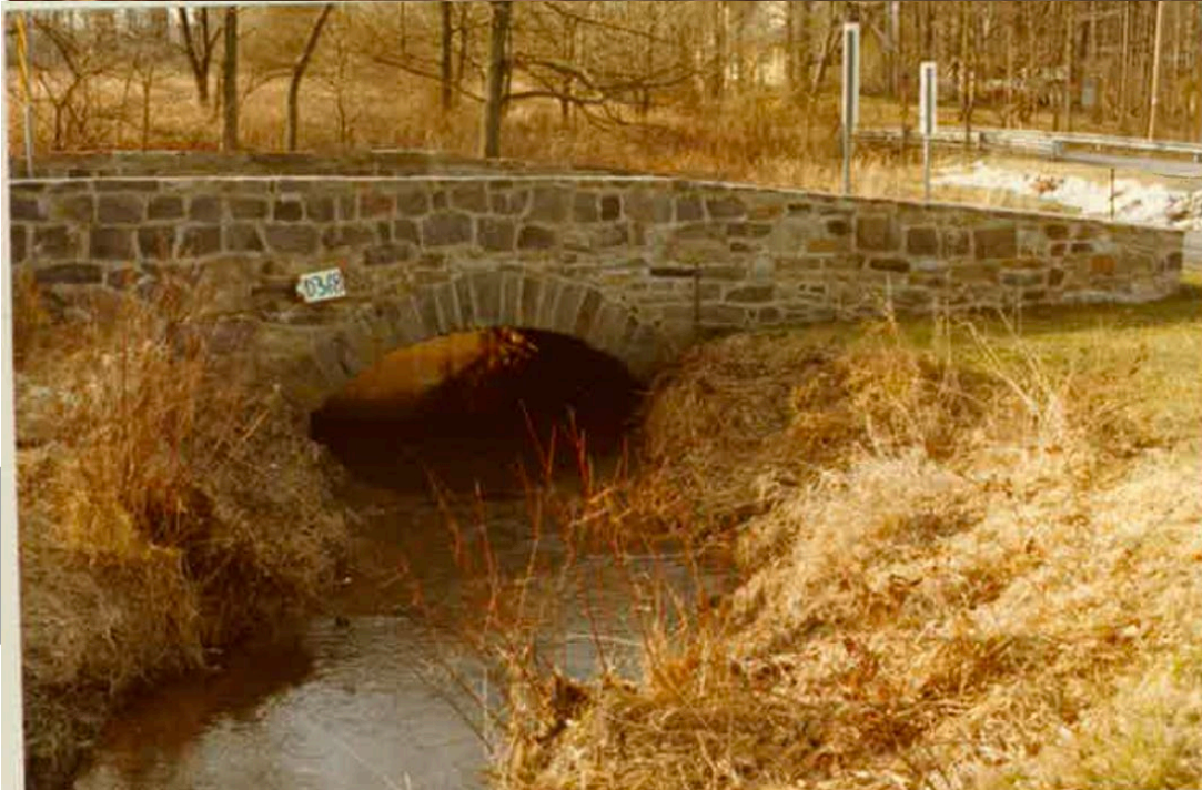
Illustration 8: circa 1980 view of the Sandbrook-Headquarters Road bridge. 8
