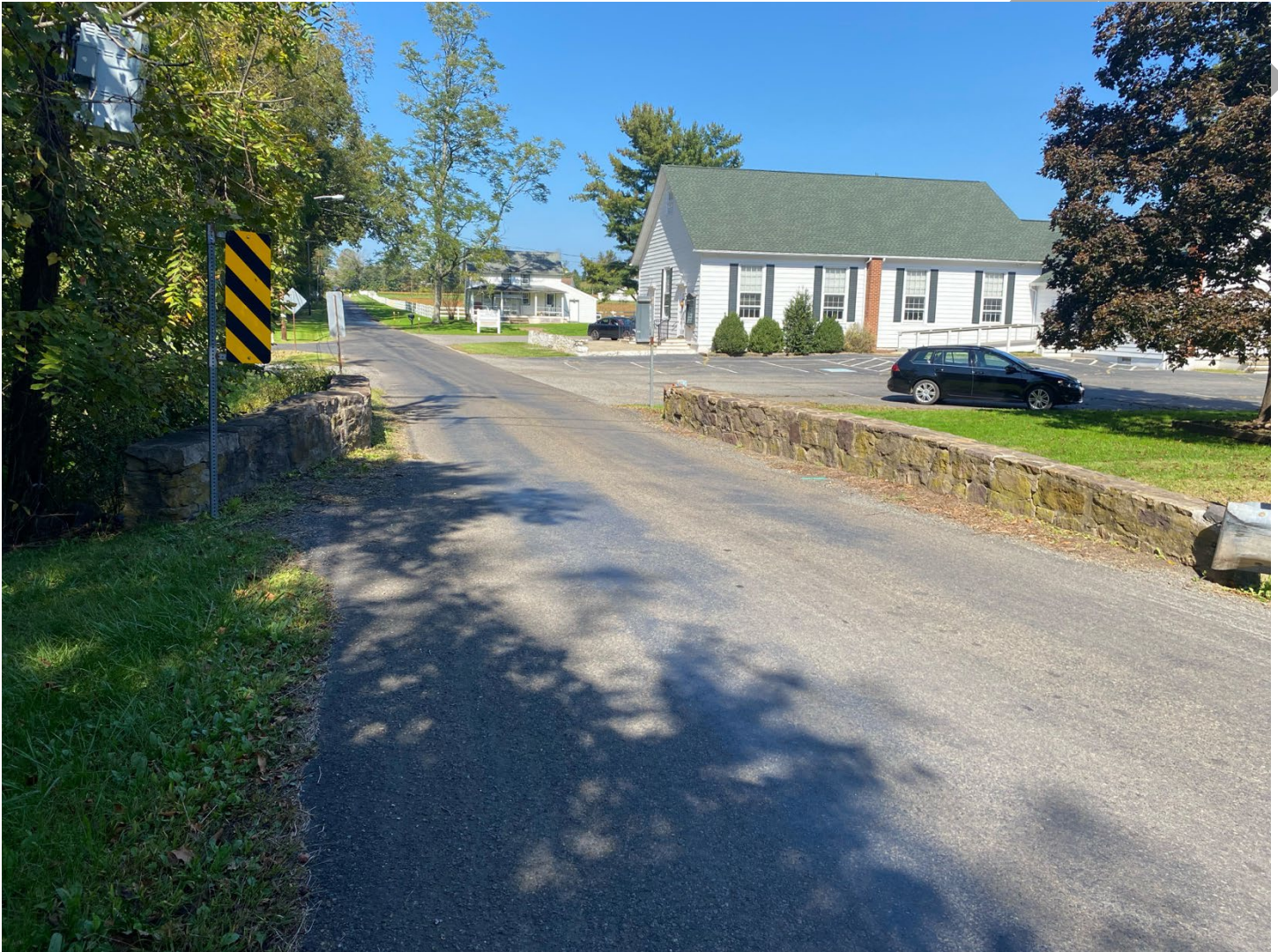
Photo 1: Overall view facing north on Sandbrook-Headquarters Road
